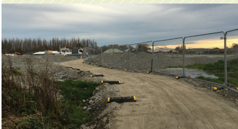
Cycle/walking detour route in the making
