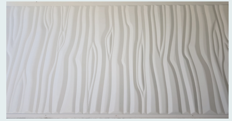
Internal wall decoration representing native bark. Together with the light white colour it provides a feeling of space and openness.
