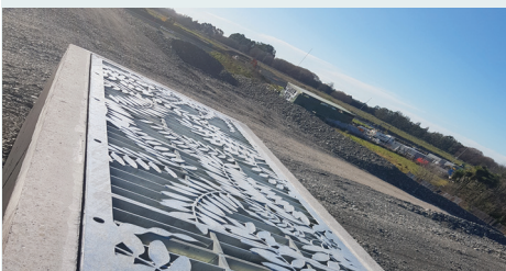
Light wells in the roof space allow for natural light to come in. The wells are decorated with shapes of native leaves and plants.
