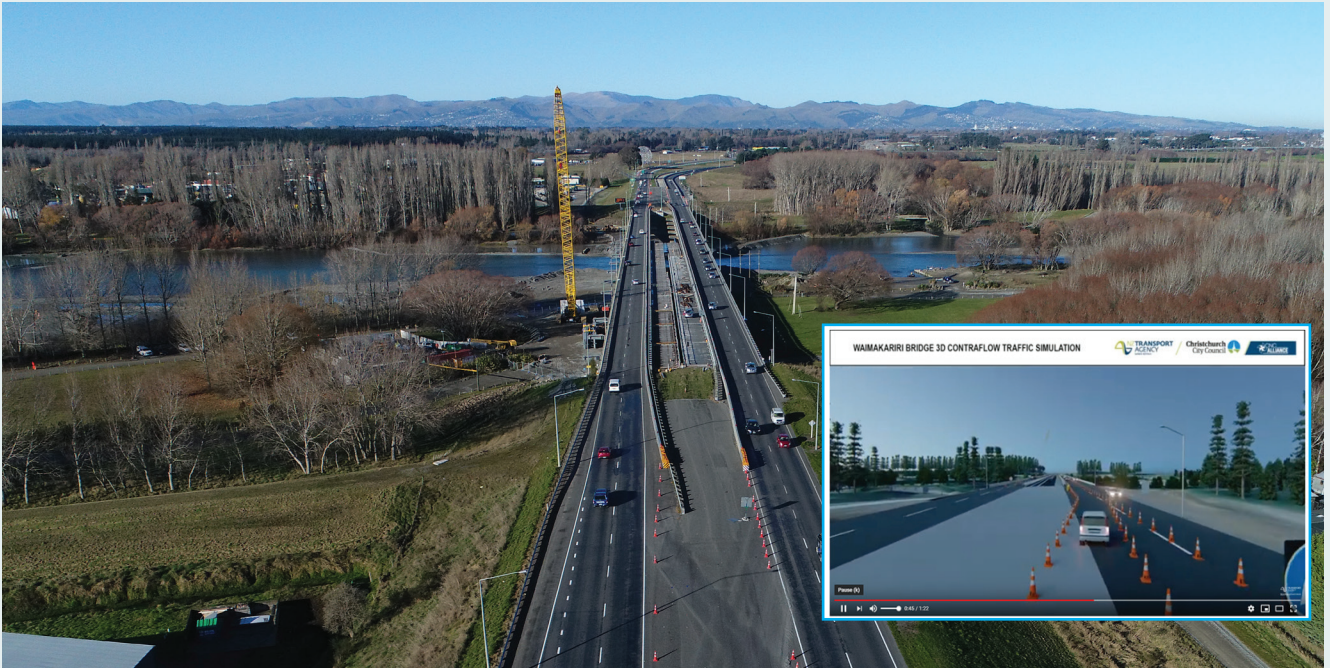
A temporary sealed section of road at the southern and northern end of the bridges accommodates the contraflow. An animated video on our website: www.nzta.govt.nz/cnc shows how the Waimakariri Bridge contraflow will work.
