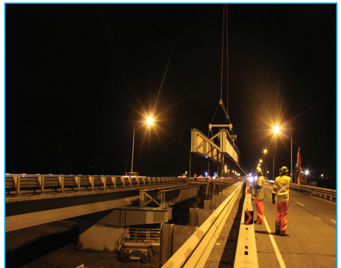
Lifting the bridge spans at night.
