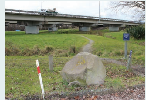
When we are working underneath and in between the two bridges we will have to close part of the walking track on the park.
