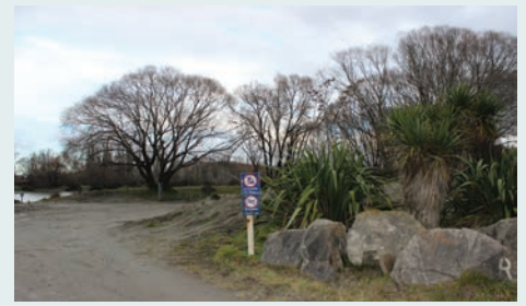
During our work we will have a temporary access road in the reserve to reach the boat ramp.
