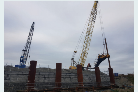
Removing the drilled out material before we add the steel reinforcement.
