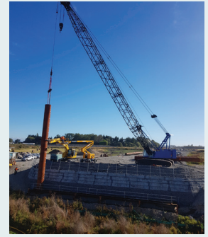
First steel casing going in.
