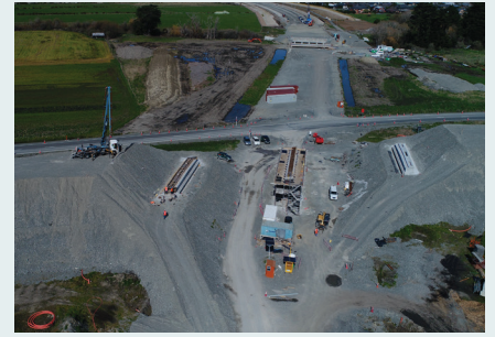
Radcliffe Road Bridge in construction.
