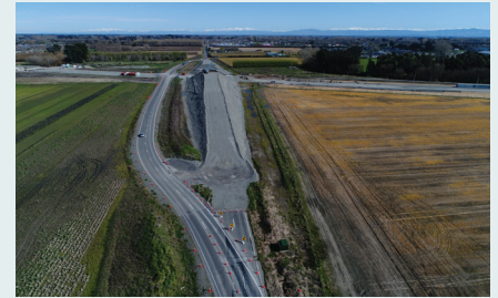
The temporary road next to the Radcliffe Road bridge abutments.
