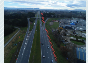
SH1 between Tram Road and the Waimakariri Bridge. Red diamond line shows our work area.
