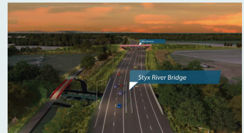
Artist's impression of the Styx River Bridge for motorists with a separate bridge for walkers and cyclists shown on the left.
