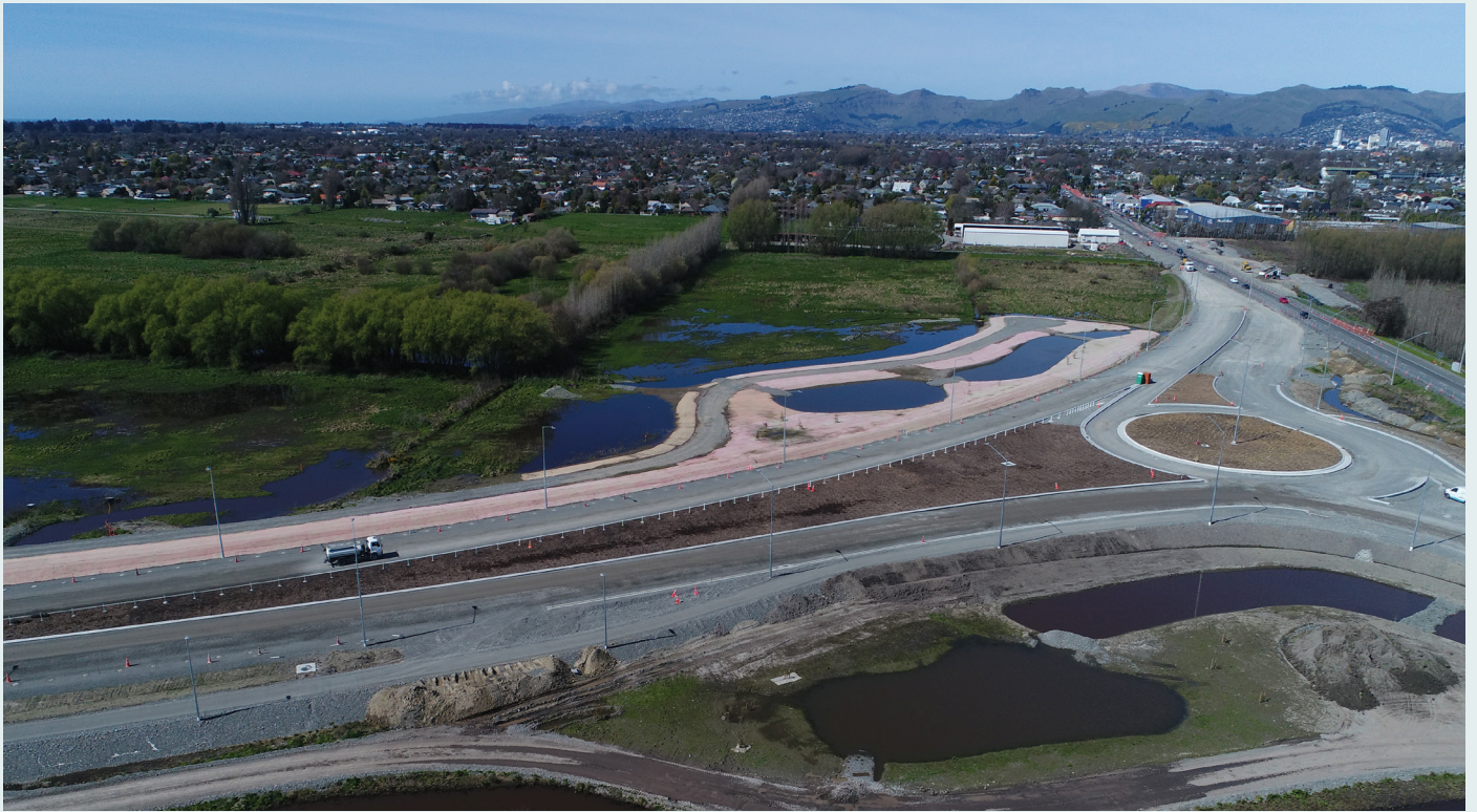
The CNC motorway goes through Cranford Basin to connect to Cranford Street via a roundabout. The speed through the Cranford basin section will reduce from 80km/h at QEII Drive to 50km/h on Cranford Street.
