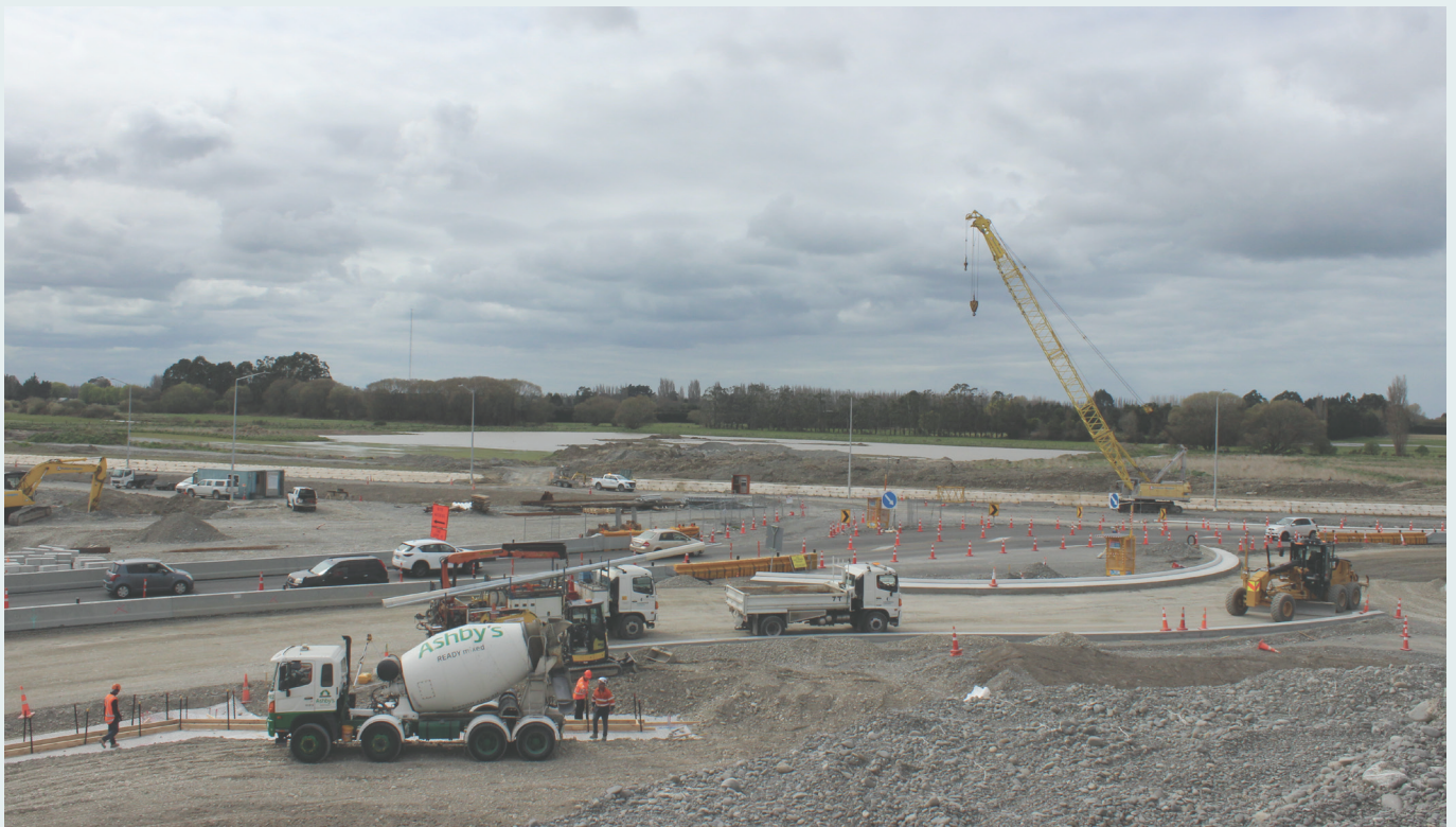
The QEII Drive interchange in construction.
