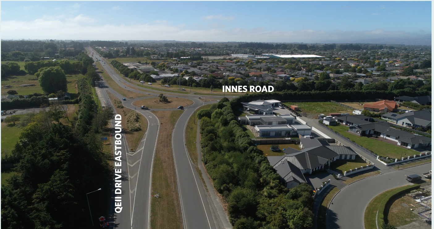
QEII Drive/Innes Road roundabout: the roundabout will be upgraded to include the two eastbound lanes on QEII Drive, an extra westbound lane on the roundabout and a slightly relocated slip lane to Innes Road.
