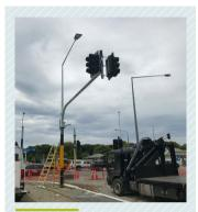
When the existing street light pole (right in the photo) has been removed, we can turn the new gantry into the right position (over the road) and turn on the new street lights and traffic signals.
