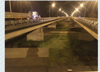
Barrier installation last week Tuesday on the northbound bridge
