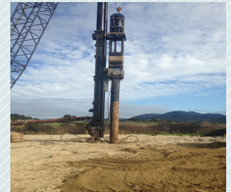
A timber piling rig in action
