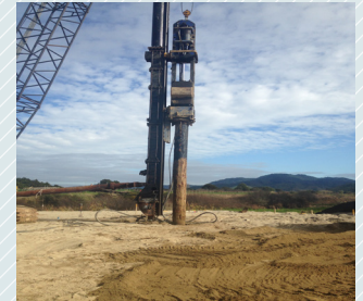
A timber piling rig in action
