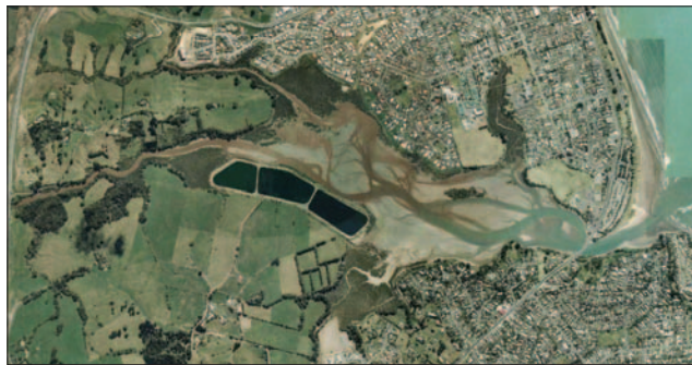
Left is the Hibiscus Coast Highway running between Orewa town and the main beach and right is the ALPURT B2 – Northern motorway extension that directs traffic around the outskirts of Orewa
