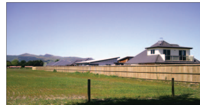
Noise barrier constructed by a developer next to proposed link road to the Christchurch Southern Motorway
