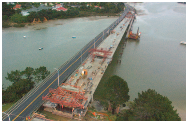
Widening of the SH18, Upper Harbour Causeway completed, June 2006
