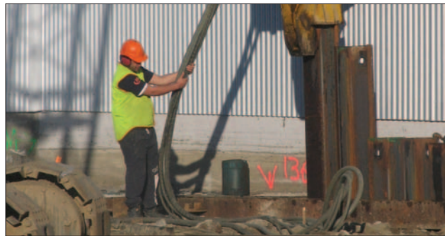
A vibrating hammer being used to drive sheet piles
