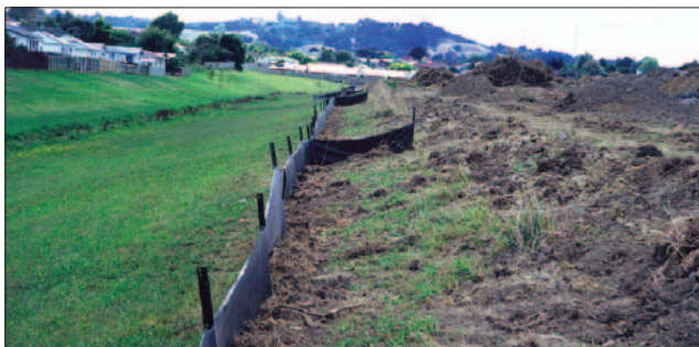
Silt fence construction (Photo in Auckland region – compliments ARC)
