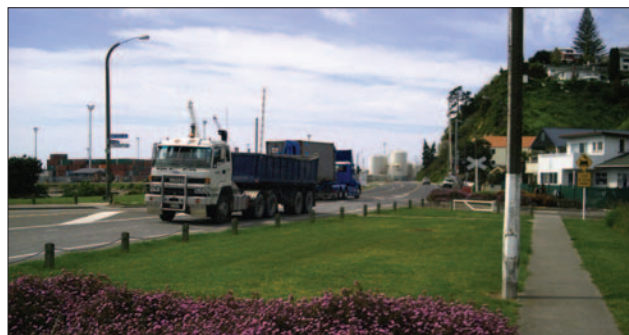
SH50 near Napier port where a replacement low-noise surface reduced traffic noise problems for residents in the area
