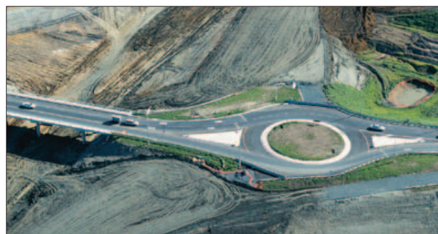
Orewa Interchange construction, ALPURT B2 Northern Motorway Extension
