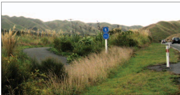
The cycle pathway along SH1 north of Plimmerton received a bronze award for Sustainability in Landscape Design from the New Zealand Institute of Landscape Architects
