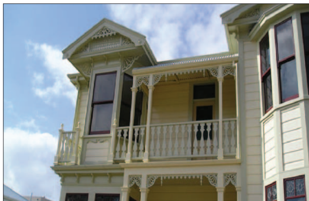
Historic house on Tonks Ave, Wellington inner city bypass
