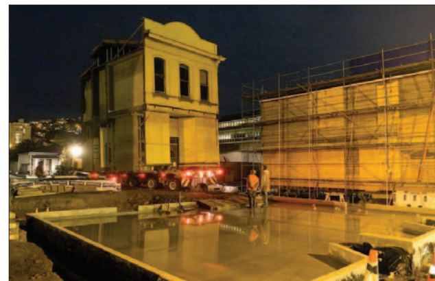
Relocation of 291 Cuba St
