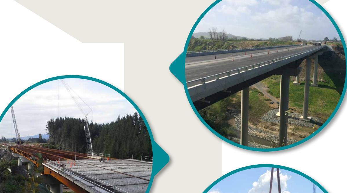
To complete the bridge, the road surface (pavement) was laid, bridge barriers attached, wire rope barrier installed and road marking painted.
