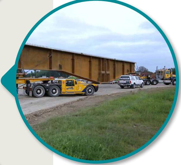
A truck and jinker transported the steel beams to site. Note the size of this beam in comparison to the vehicle in the middle.
