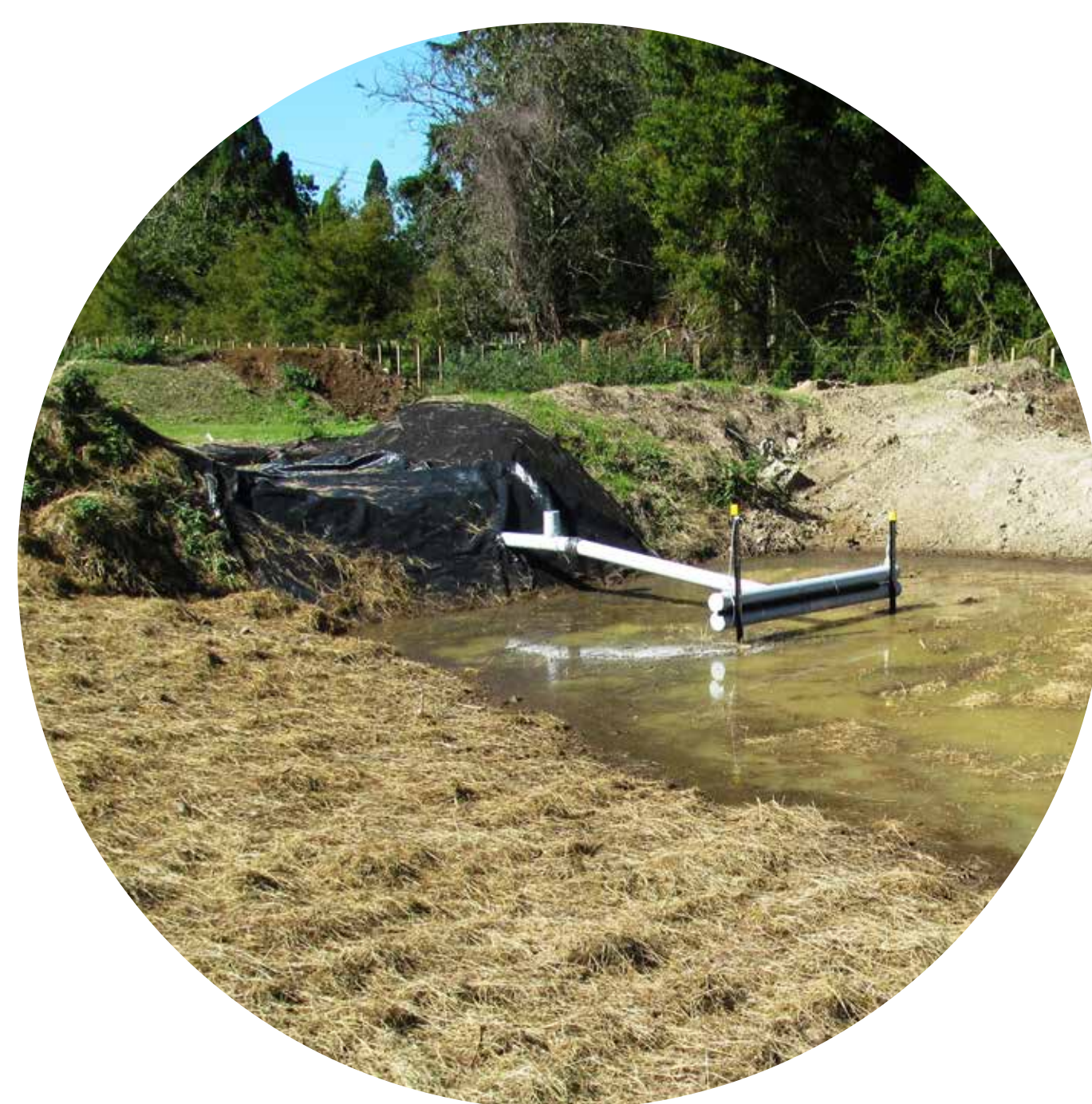
Erosion and sediment control
