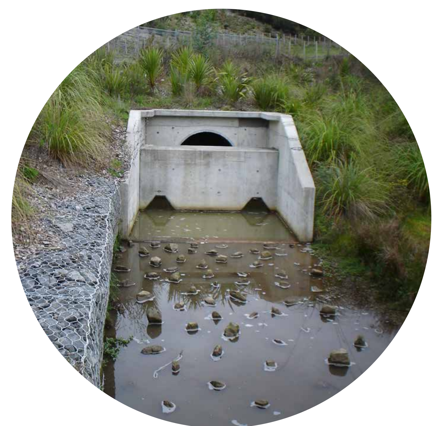
Culvert water diffuser
