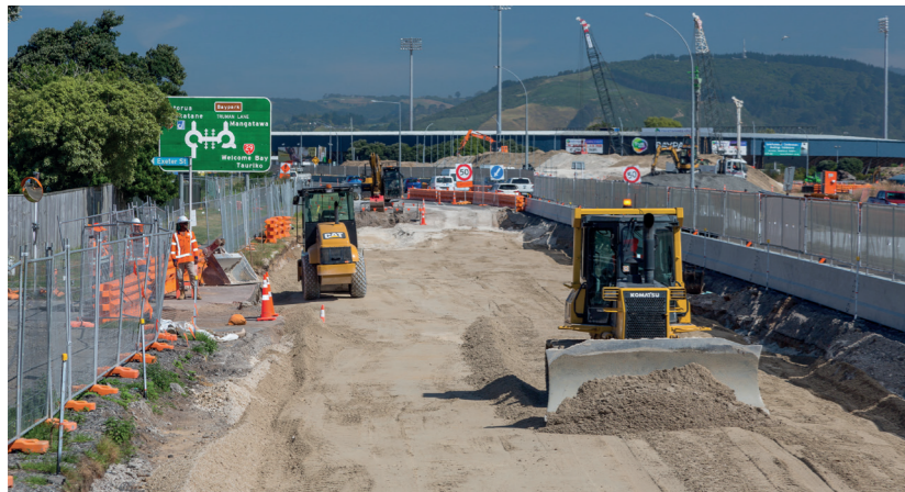
Works continue on SH2 near Te Maunga.
