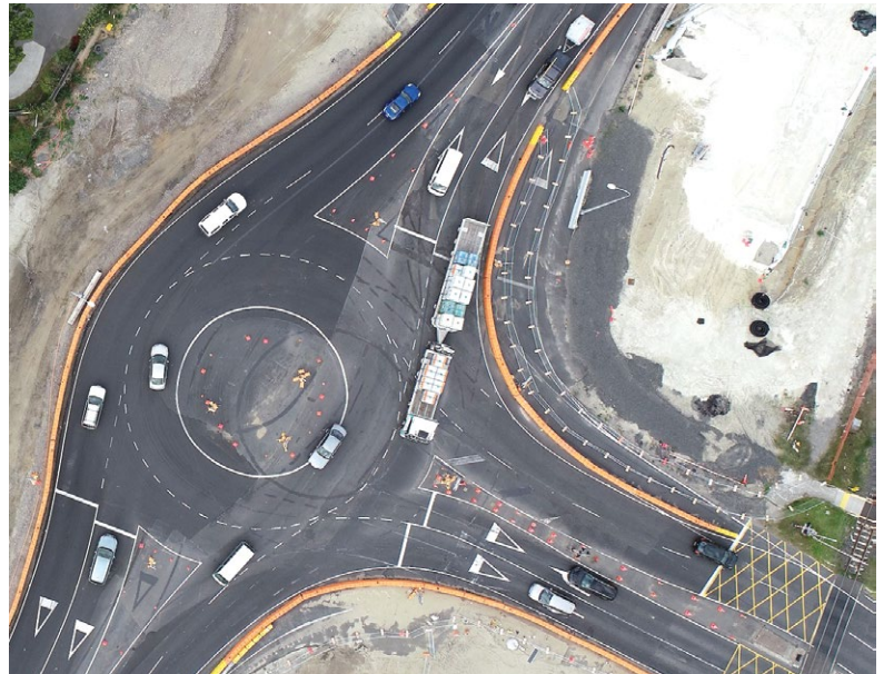
An aerial view of the existing Te Maunga roundabout.
