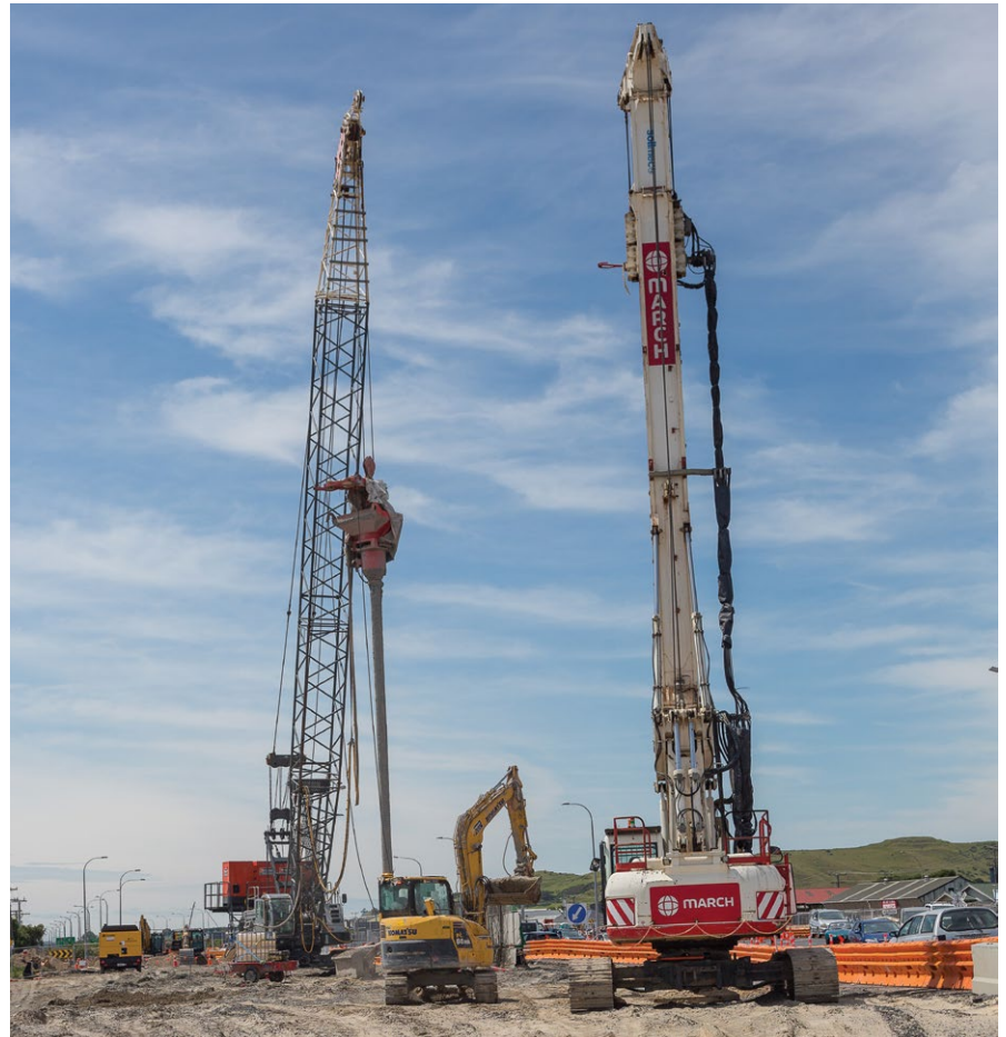
Stone column rigs.
