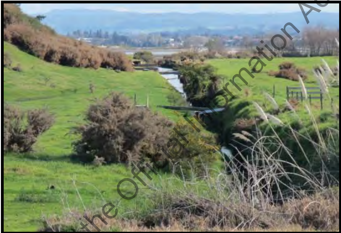
Figure 8 Stormwater drain discharging into Waipū Estuary, adjacent to Omanu Urupa
