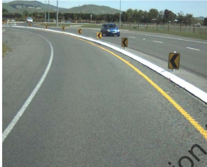
Figure 4 – Example of PW-67 chevrons on a median approaching a roundabout.
