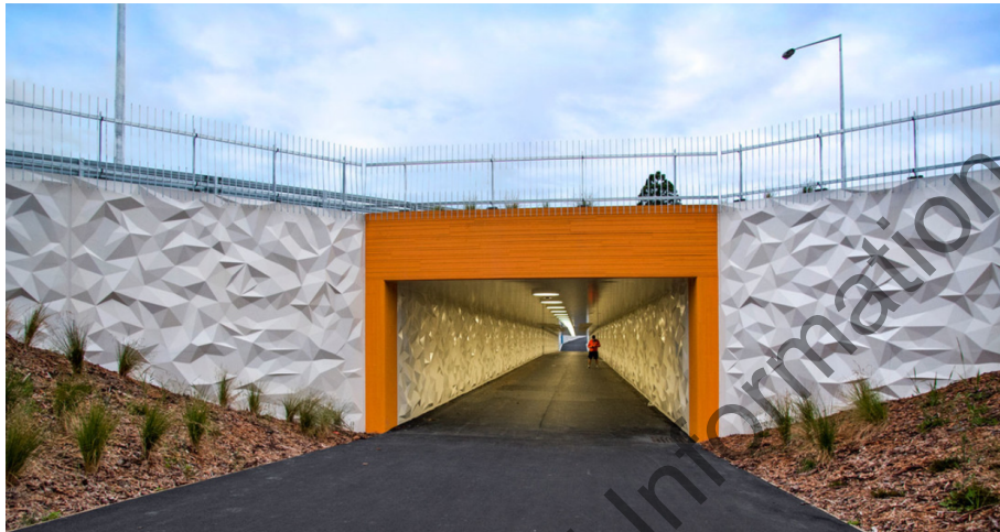
Figure 6: Photo of SH1 Russley Road/Harewood Road underpass
