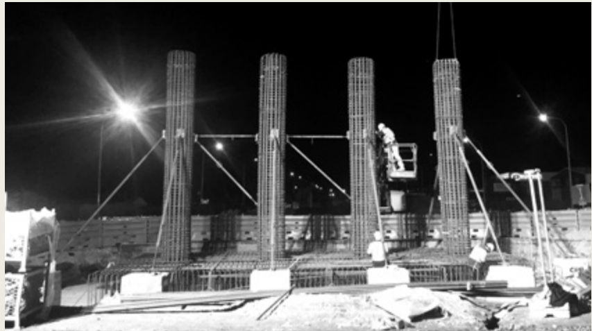
The first Bayfair flyover pier under construction
