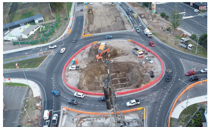
Aerial view of the ground improvement works underway earlier this year
