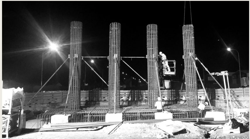
The first Bayfair flyover pier under construction
