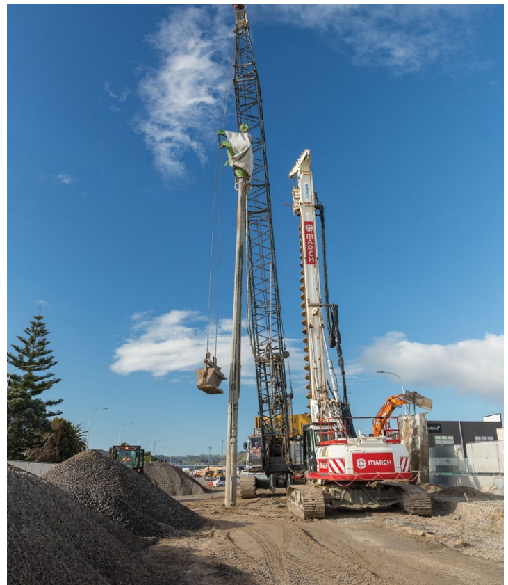
More than 850 stone columns have been installed in the work area east of the Bayfair roundabout. The stone columns in this area will help support the weight of the flyover that will be built on top. The stone column rig has now returned to near the Te Maunga roundabout.
