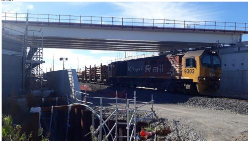
Twelve beams were craned into position over three nights in February, completing the structure on which the bridge's deck and pavement will be constructed. The reinforced concrete beams were manufactured in Te Puke and weigh approximately 55T each. They were installed by a single 450T crane following coordination with Tauranga Airport and KiwiRail about plane and train movements in the area.
