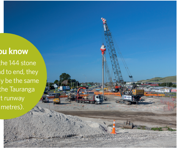
Stone column work is continuing near Te Maunga and Baypark.
