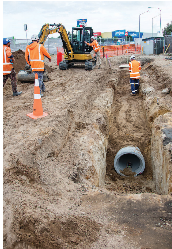
Stormwater drainage installation and utility service relocation on Matapihi Road
