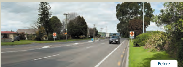
Maunganui Road looking east towards SH29/2 interchange
