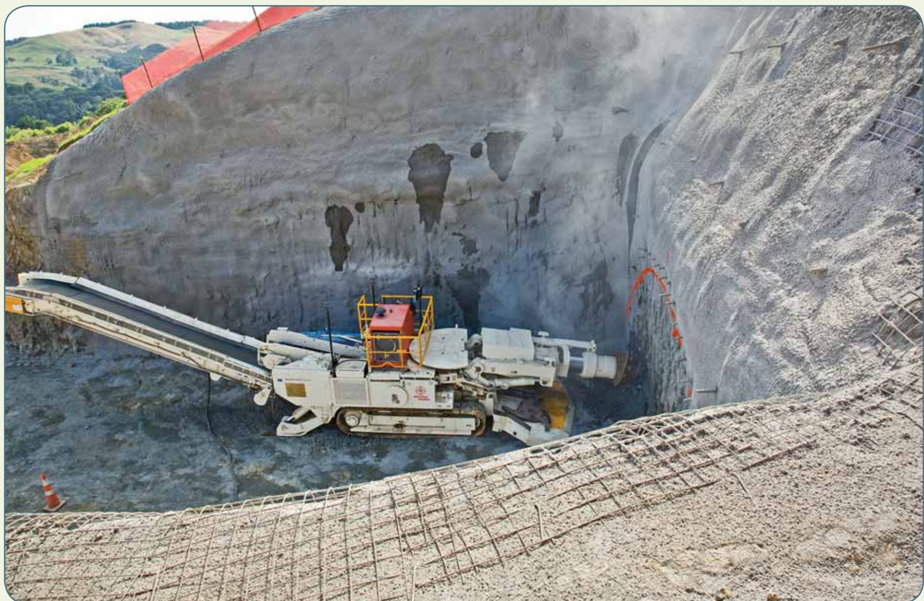
Photo of tunnel construction from WTA scoping report. The tunnel will be bored for most of its length. A small section of cut-and-cover tunnel is likely to be needed at the Hataitai entrance.
