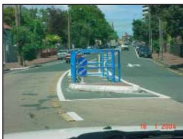
Figure 7-28: Typical Kea Crossing Configuration 1
