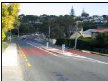
Figure 7-28: Typical Kea Crossing Configuration 1
