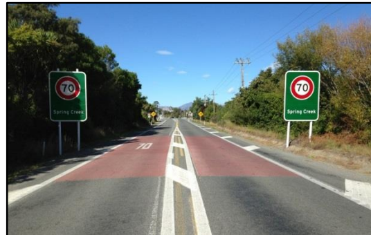
Figure 3: North speed threshold looking south
