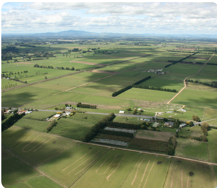
Collins Road area looking south-east
