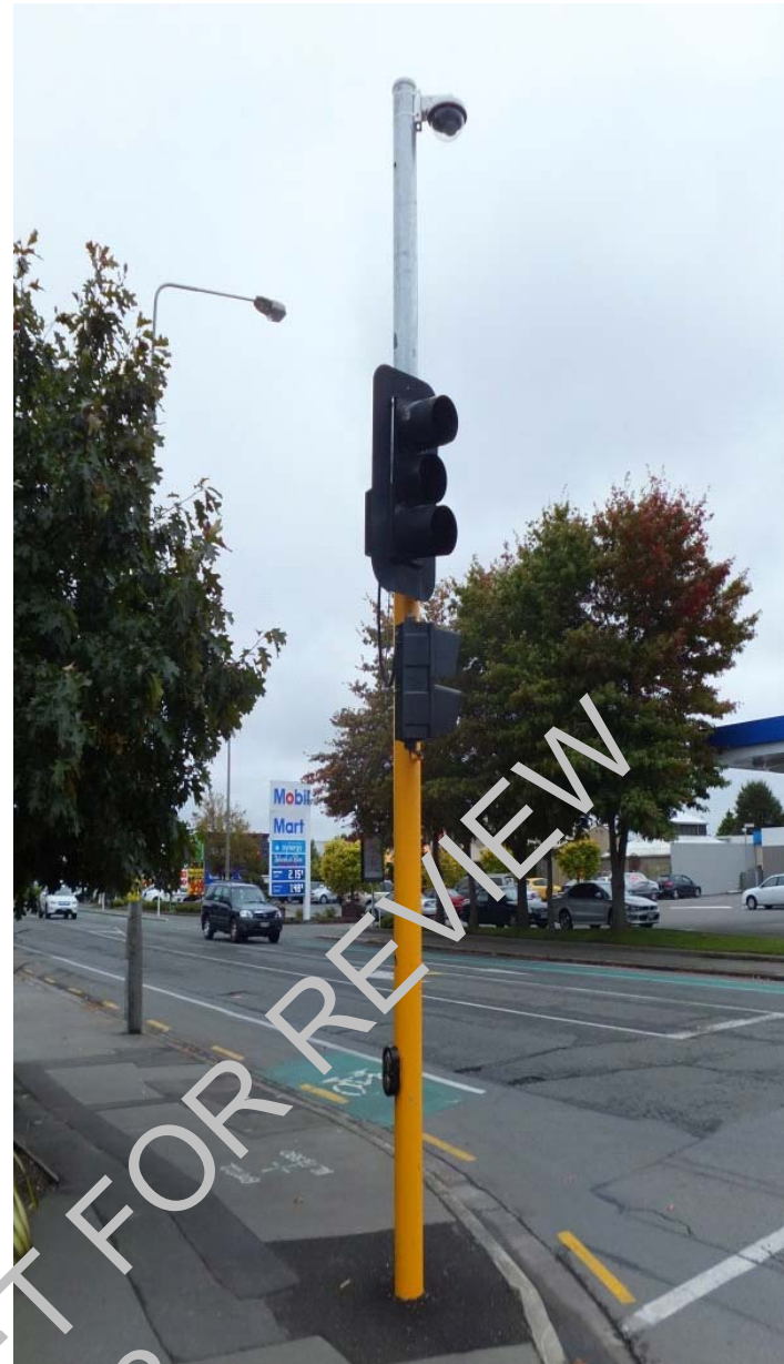
Spunlite Type 2 Combined CCTV / Traffic Signal Pole
