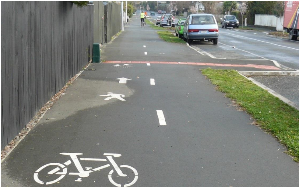
Figure 5.18 Shared Path, Toi Toi Street, Nelson
