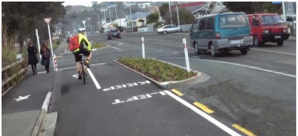
Figure 6.3 Intersection of a bi-directional facility and a side road, St Vincent Street, Nelson
