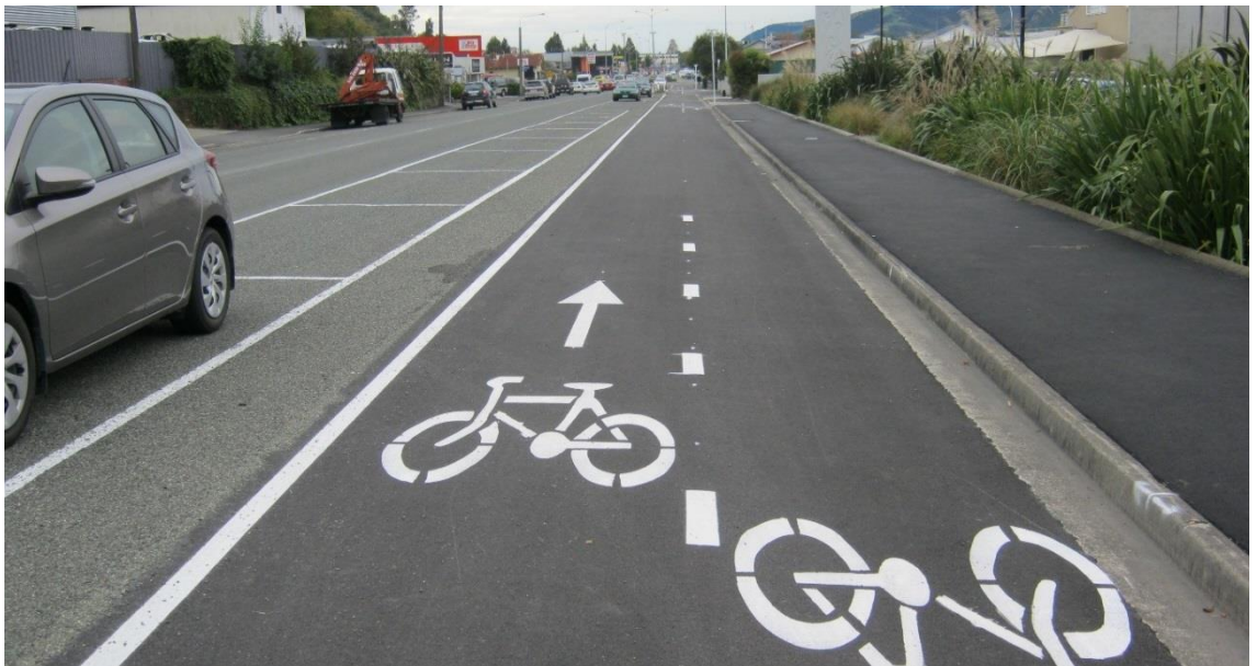
Figure 5.15 Two way Protected Bicycle Lane, St Vincent Street, Nelson (prior to the addition of a separator)
