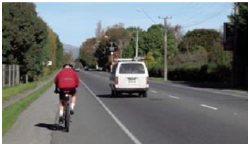
Figure 5.12 Photo of Sealed Shoulder (Source: CNPRG Chapter 6)
