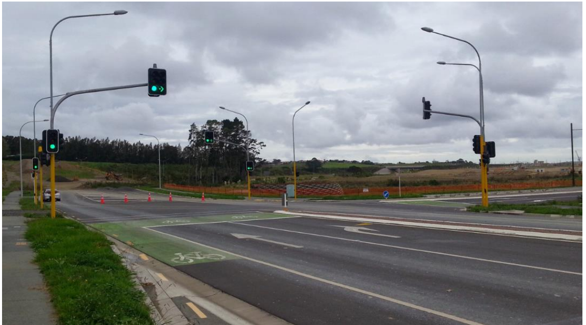
Figure 6.5 An example of a typical signalised T-intersection with cycle facilities (Northside Dr/Tahi Rd Auckland)
