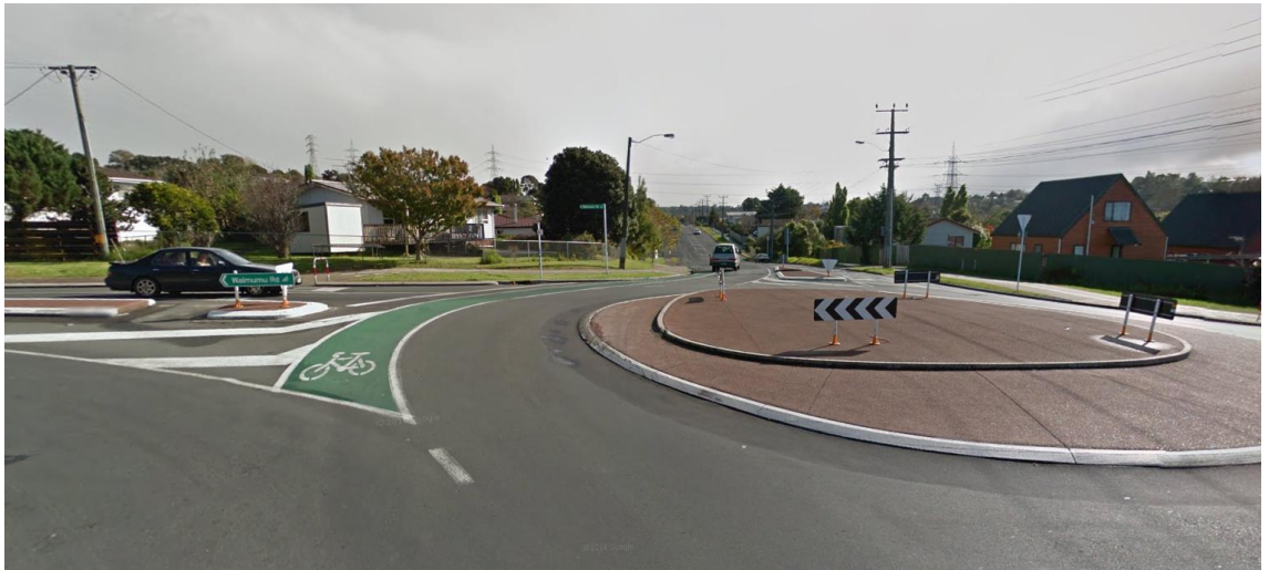
Figure 6.9 Cycle lane in Triangle/Waimumu Roundabout, Auckland
