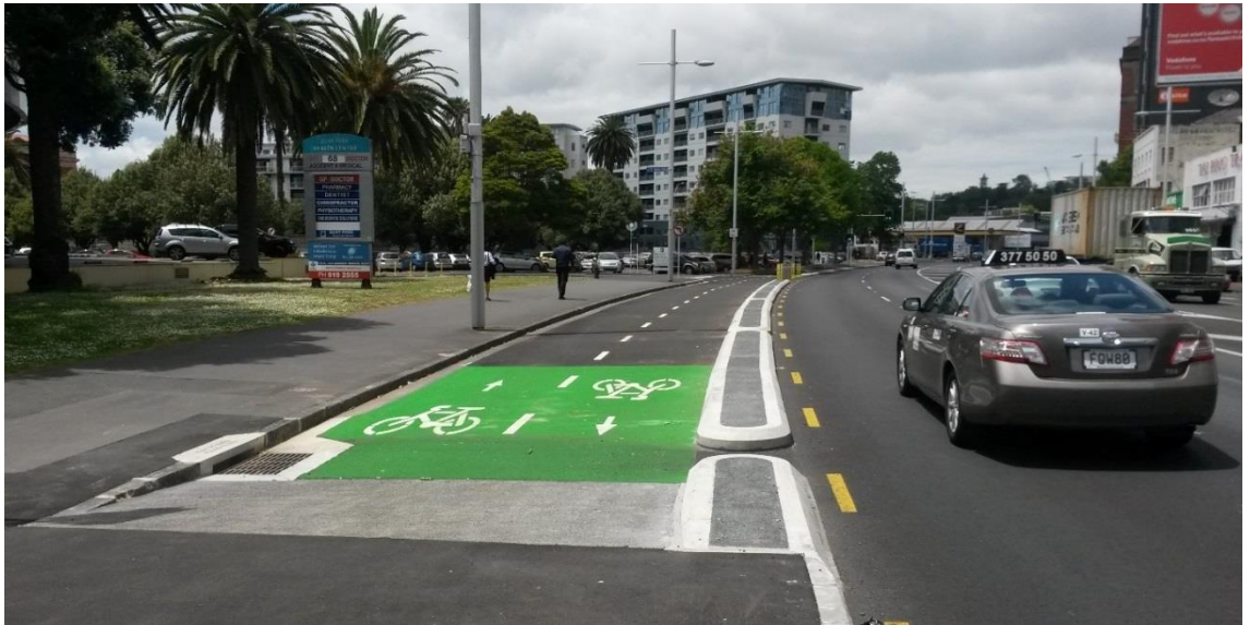
Figure 5.14 Two-way Protected Bicycle Lane, Beach Road, Auckland
