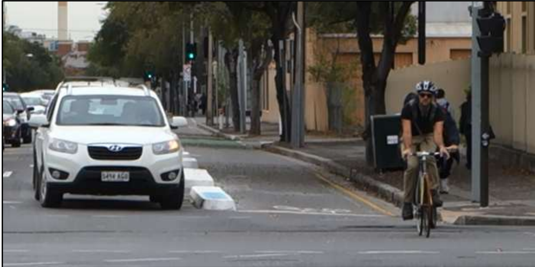
Figure 1-2: Potential for conflict between left turning vehicle and cyclist travelling straight from separated cycleway (Adelaide, Australia)
