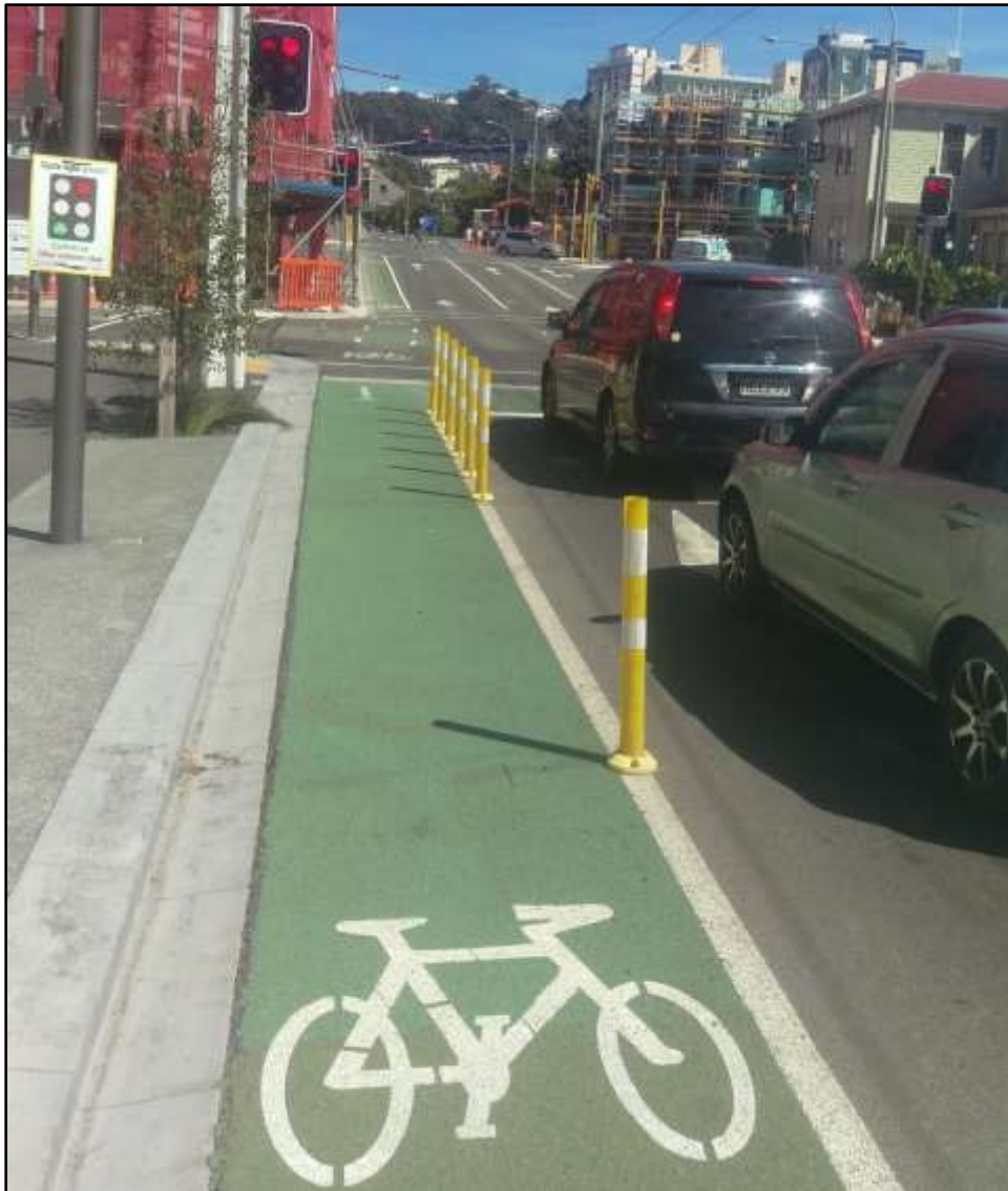
Figure 1-1: Conflict between left turning vehicles and cyclists travelling straight from kerbside separated cycleway (Wellington)
