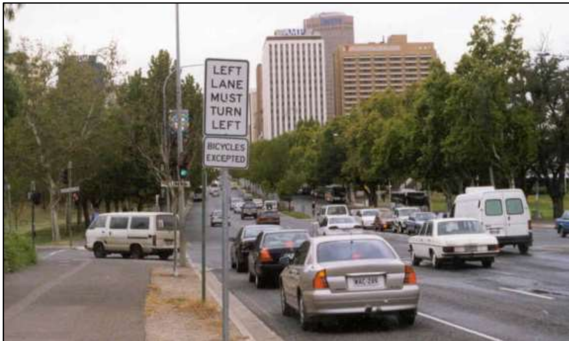
Figure 3-7: Example of a signed left-turn lane where cyclists can go straight, Melbourne, Australia
