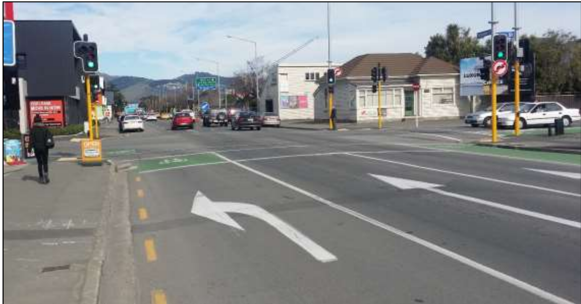
Figure 3-5: Advanced stop box in front of left-turn lane, Christchurch
