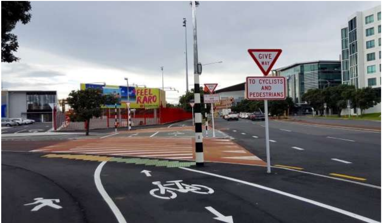
Figure 2-10: Recently installed shared path crossing with raised platform, Quay St, Auckland - legally ambiguous but probably works adequately
