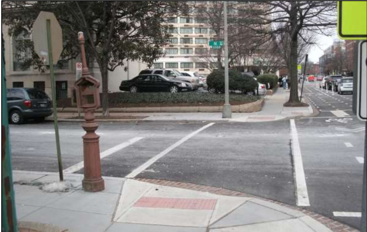
Figure 2-7: Parallel line crosswalk markings at a STOP-controlled intersection, Washington DC, USA
