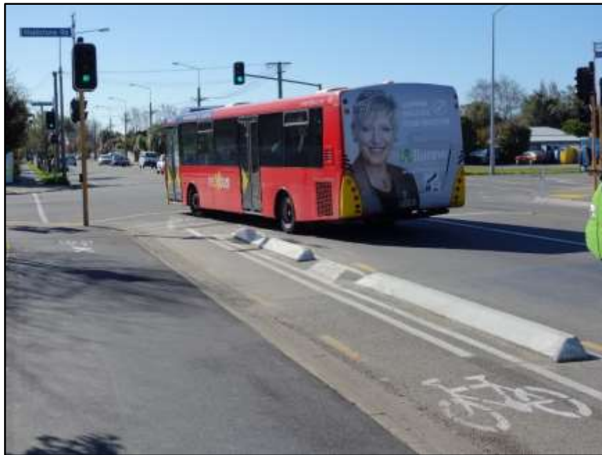
Figure 1-3: Potential for conflict between left turning (heavy) vehicle and cyclist travelling straight from separated cycleway (Christchurch)
