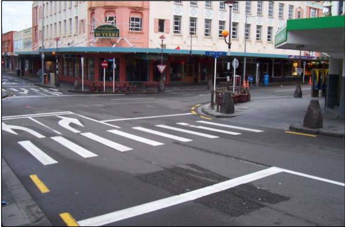
Figure 2-9: An example of a zebra crossing, slightly set back from the intersection, New Plymouth
