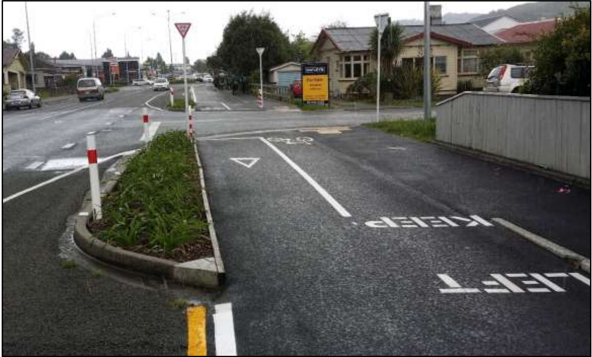
Figure 1-4: Two-way separated cycleway (Nelson) with priority ceded to side-road
