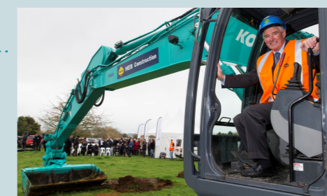
Waipa Mayor Allan Livingston turns the first sod.
