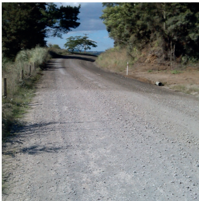
Application of magnesium chloride to Mataraua Road
