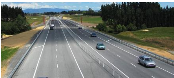
Figure 2.4: State Highway 1 Waikato Expressway near Ngaruawahia
