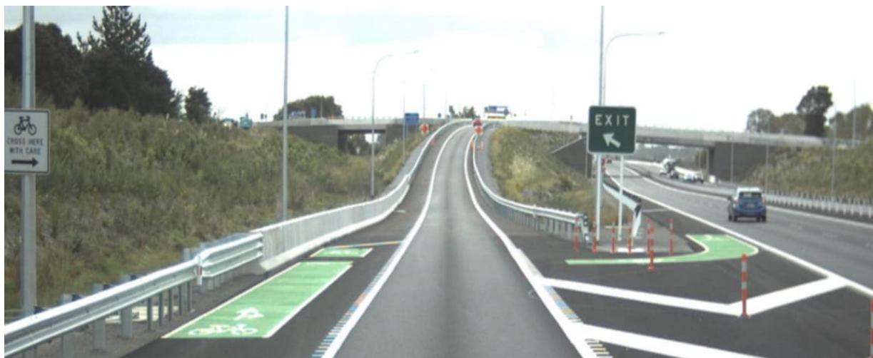
Figure 2: On road cycling facilities at northern end of the alignment
