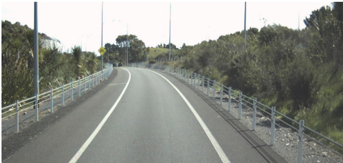
Figure 2: Southbound On-Ramp at Te Moana Road at lower elevation to mainline SH-1 reducing merge sight distance
