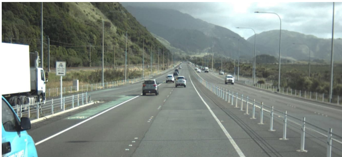
Figure 1: On road cycling facilities at southern end of the alignment (SB direction)
