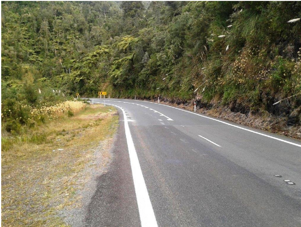
These innovative lane markings are being trialled on the entry to five deceptive curves on the pilot route in Southern Coromandel (Kopu/Whangamata/Waihi/Paeroa/Kopu).
