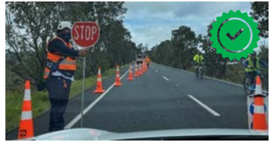
Example of a stop/go operation having a specific phase for cyclists – separating their safe travel in a single lane environment by time (from vehicles). Image Credit xlii: Betty Mitrova.
