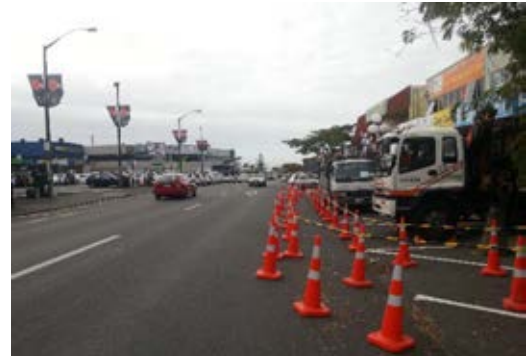
Delineation serves to channel different types of road users with a primary purpose of being visible. Image Credit Ixxix: Parallax.
