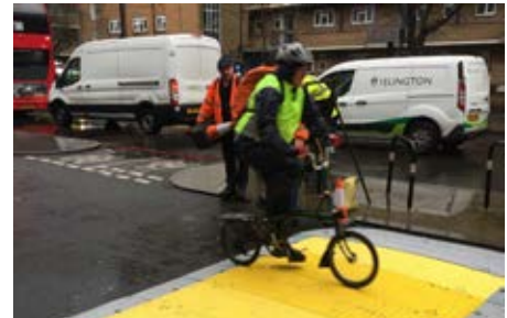
Some excavation covers are rated for vehicle and VRU use. Image Credit lxxxiii: Transport for London.
