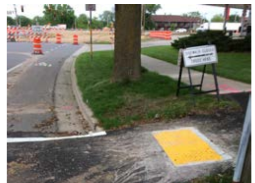
Tactile Ground Surface Indicators are an important measure for the safety of pedestrians, even at temporary crossing points. They should be considered in accordance with best local practice. Image Credit c: UW-TOPS Lab.
