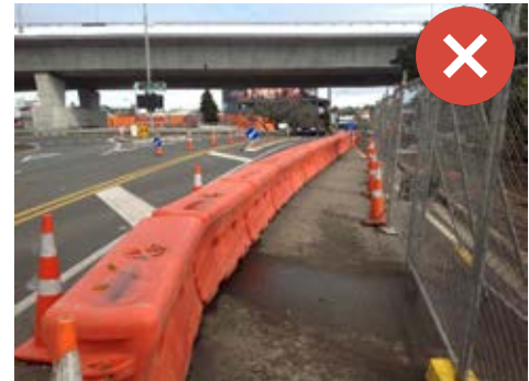
Pedestrians should not be put into the deflection zone of a barrier system. Image Credit cxi: Parallaxx.
