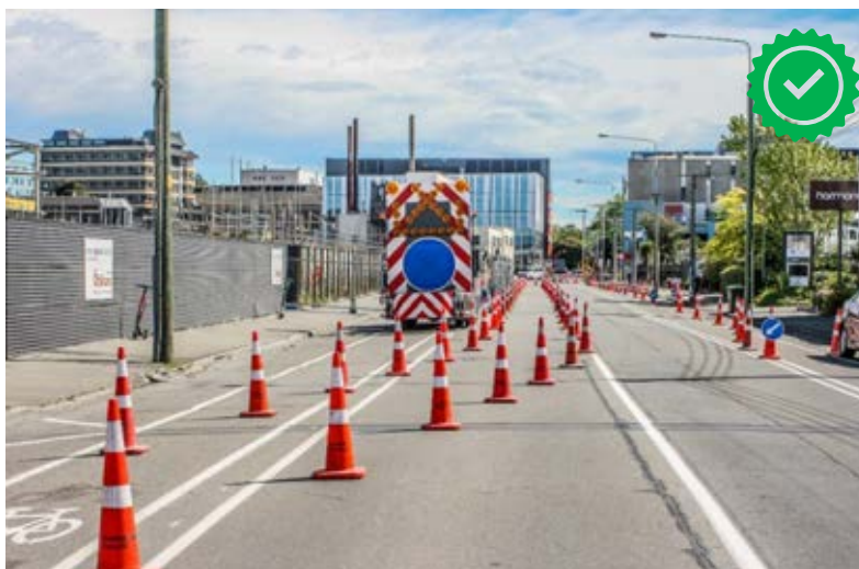
This example shows a clear and well aligned temporary cycle lane diversion. One improvement would be adding a method to prevent cyclists riding through the cones (especially at the diversion location). Image Credit xlv: Whites Traffic Management.
