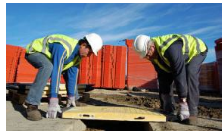
Some excavation covers can be heavy, therefore installation and removal using mechanical means is preferred. Image Credit lxxxiv: Oxford Plastics
