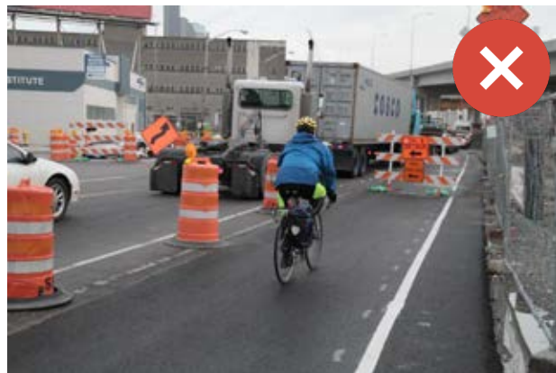
Cyclist detour with no clear safe arrangement with the nearest traffic lane at the point of detour. Image Credit li: Washington State Department of Transportation.
