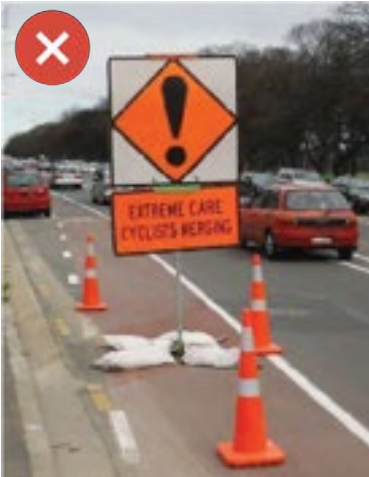
Advanced warning can help inform drivers and VRUs about upcoming hazards. Make sure not to place signs where they become a hazard themselves. Image Credit Ixxiv: Christchurch City Council.
