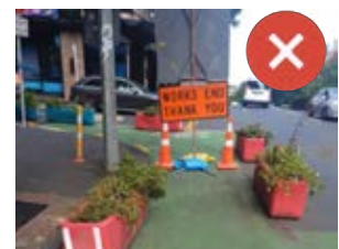
Sign placement is a key consideration. Signs can increase risk when they block or obstruct VRU paths. Image Credit xcv: UltimeciaNZ via Twitter.
