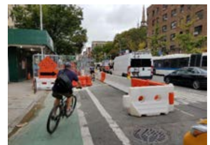
Temporary Road Safety Barriers can serve as channelisation devices too – giving clear path for where cyclists should travel. Neither cyclists nor pedestrians should be permitted to travel in the deflection zone of the barrier. Image Credit cxii: New York Department of Transport.
