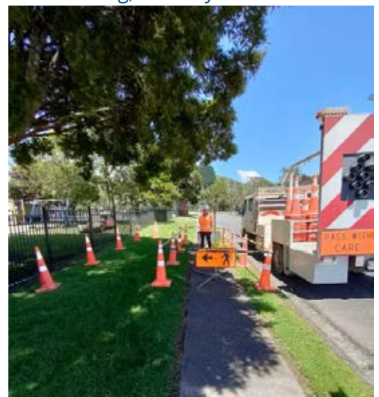
Whilst this grass area might be stable in good weather and with light use – that will quickly change after some use or rain, creating an unsafe surface for many users – especially those with mobility challenges. Image Credit Ixiv: Betty Mitrova.
