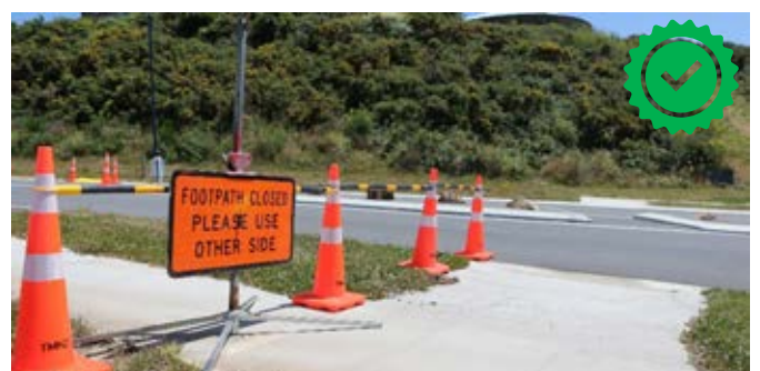
Example of footpath closure (using other side) utilising an existing pedestrian refuge. Image Credit xlix: Danny Wood.
