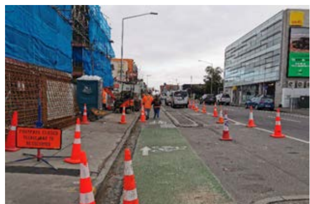
Visually impaired users especially benefit from being escorted through road works due to the highly challenging nature of TTM and the number of hazards. Image Credit lxxii: Carina Duke.
