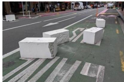
**Figure 4: concrete separators dislodged, Auckland**
