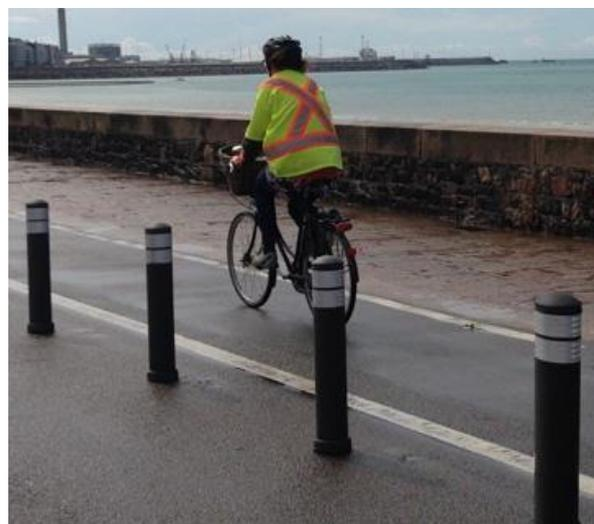
**Figure 17: delineator bollards not placed on a lane line**
