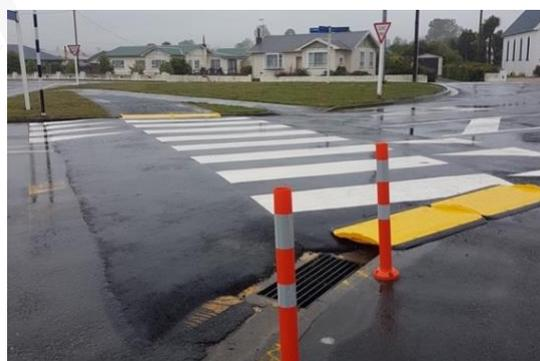
**Figure 26: temporary asphalt zebra platform with 1:20 gradient, Takaka (P. Kortegast)**
