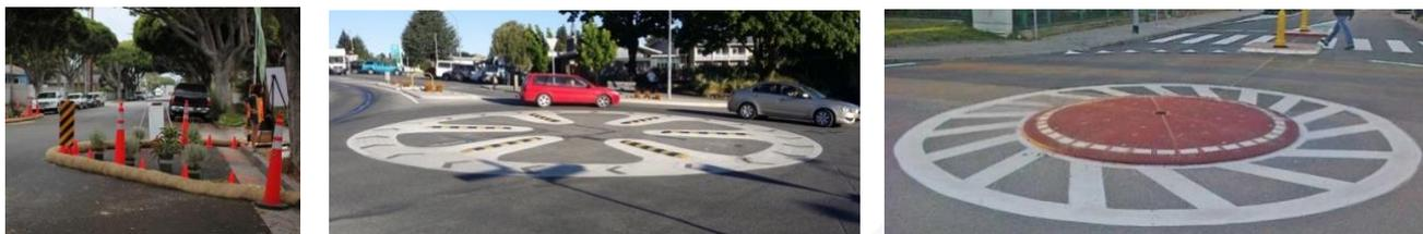
**Figure 20: demonstration kerb extensions using hay rolls (left), interim roundabouts using rubber humps (centre) or rubber islands (right)**
