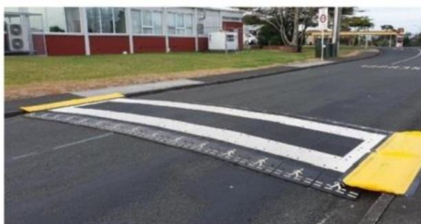
**Figure 23: a platform with fillers at the kerb; markings not compliant with TCD Rule (O. McLean)**
