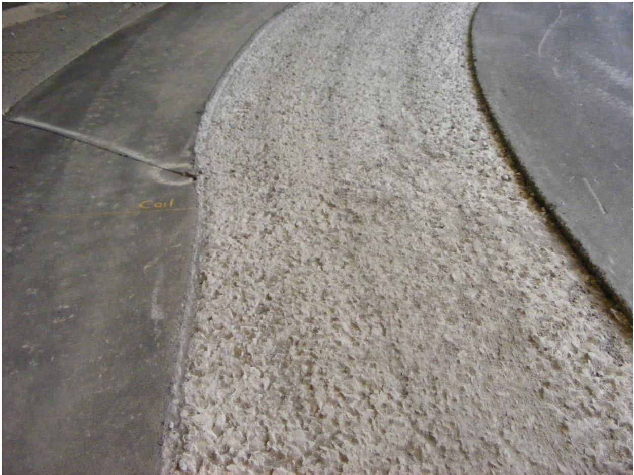
Figure 32 Milled out Dense Graded Asphalt
