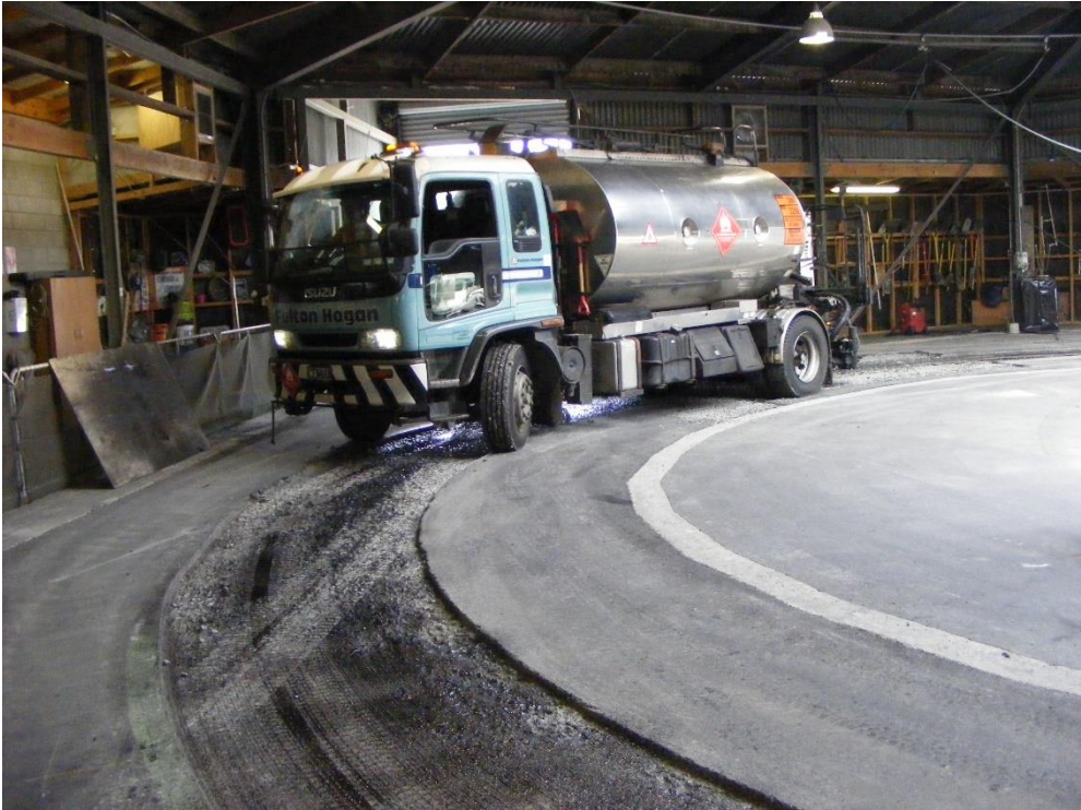
Figure 34 Membrane Chipsealing
