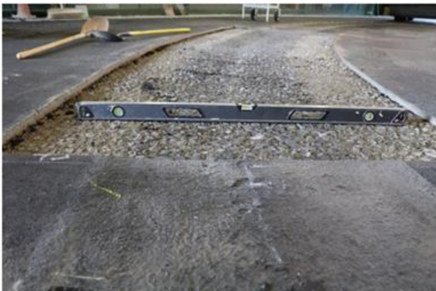
Figure 27 Repairs during loading
