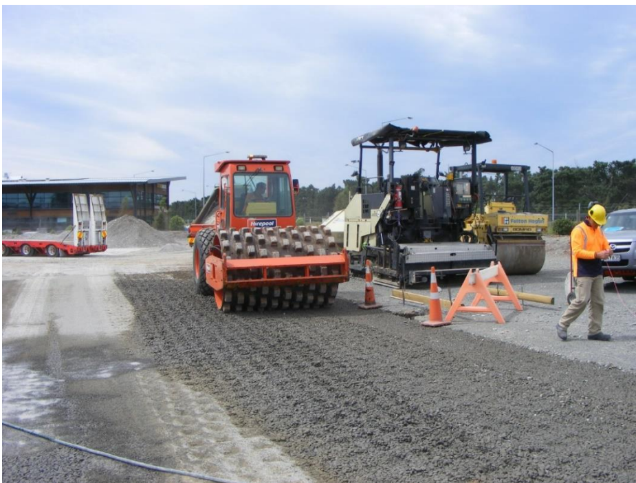
Figure 13 Hi-Lab 40 Primary Rolling with Padfoot
