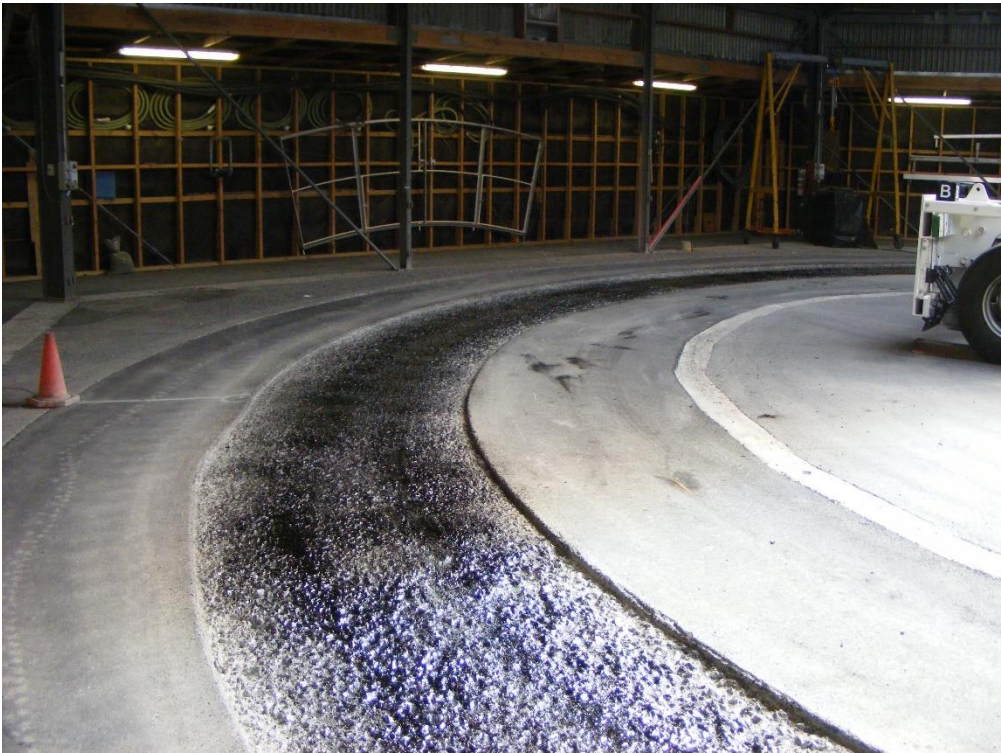
Figure 33 Priming of milled surface
