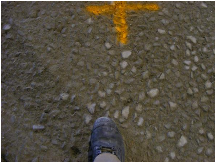
Figure 16 Hi-Lab 40 finished surface prior to sealing
