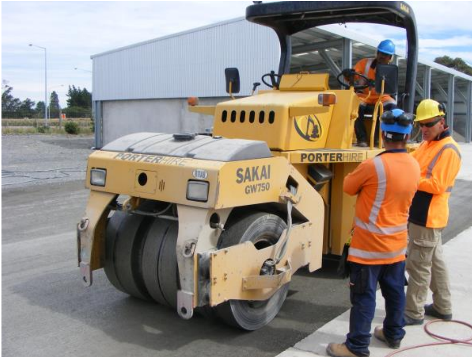
Figure 14 Hi-Lab 40 Secondary Rolling with Pap 7 to choke the surface
