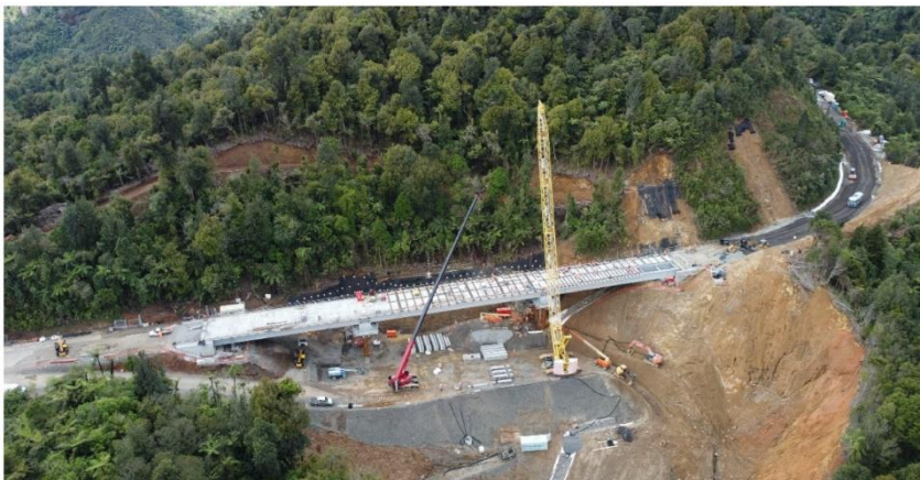
Figure 15. Repair of the SH25A
