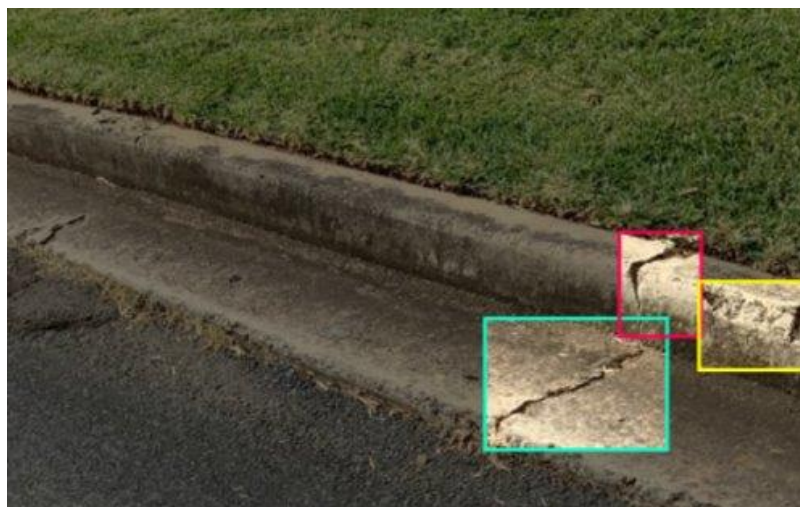
Figure 18. A pilot study by Beca used AI to detect cracks on roads.
