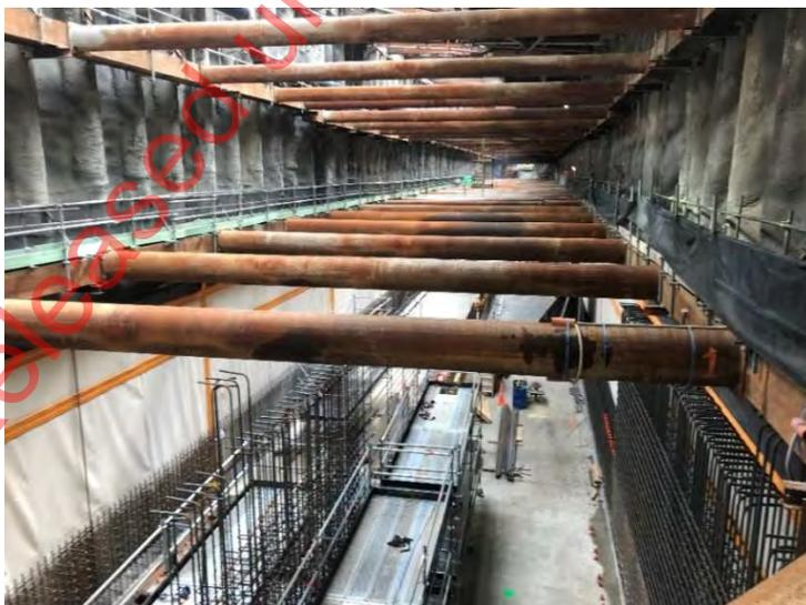
Figure 5. Cut and Cover Tunnel Construction
