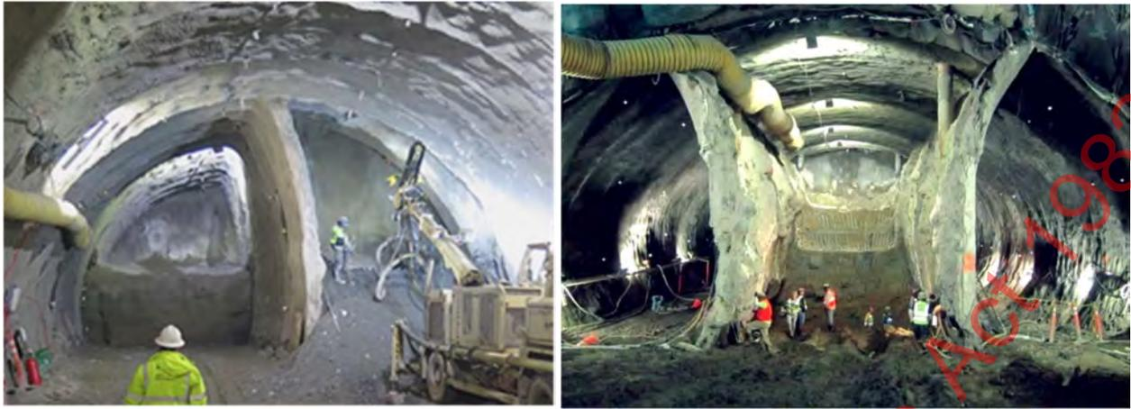
Figure 15. Examples of SEM excavation
