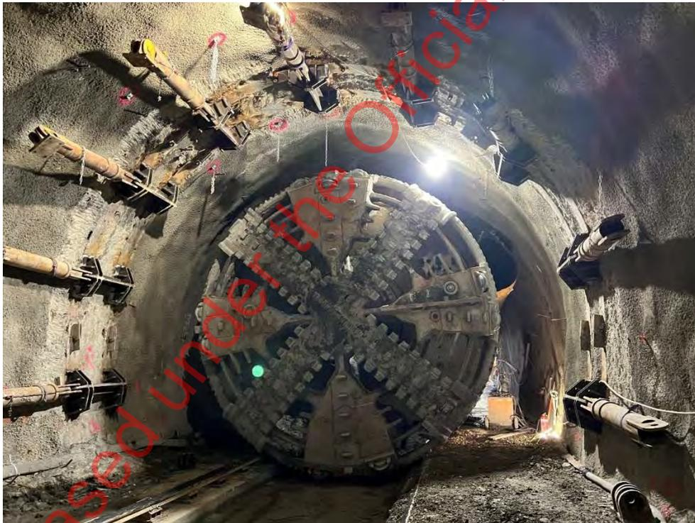
Figure 16. TBM transfer through a mined cavern, City Rail Link, Auckland
