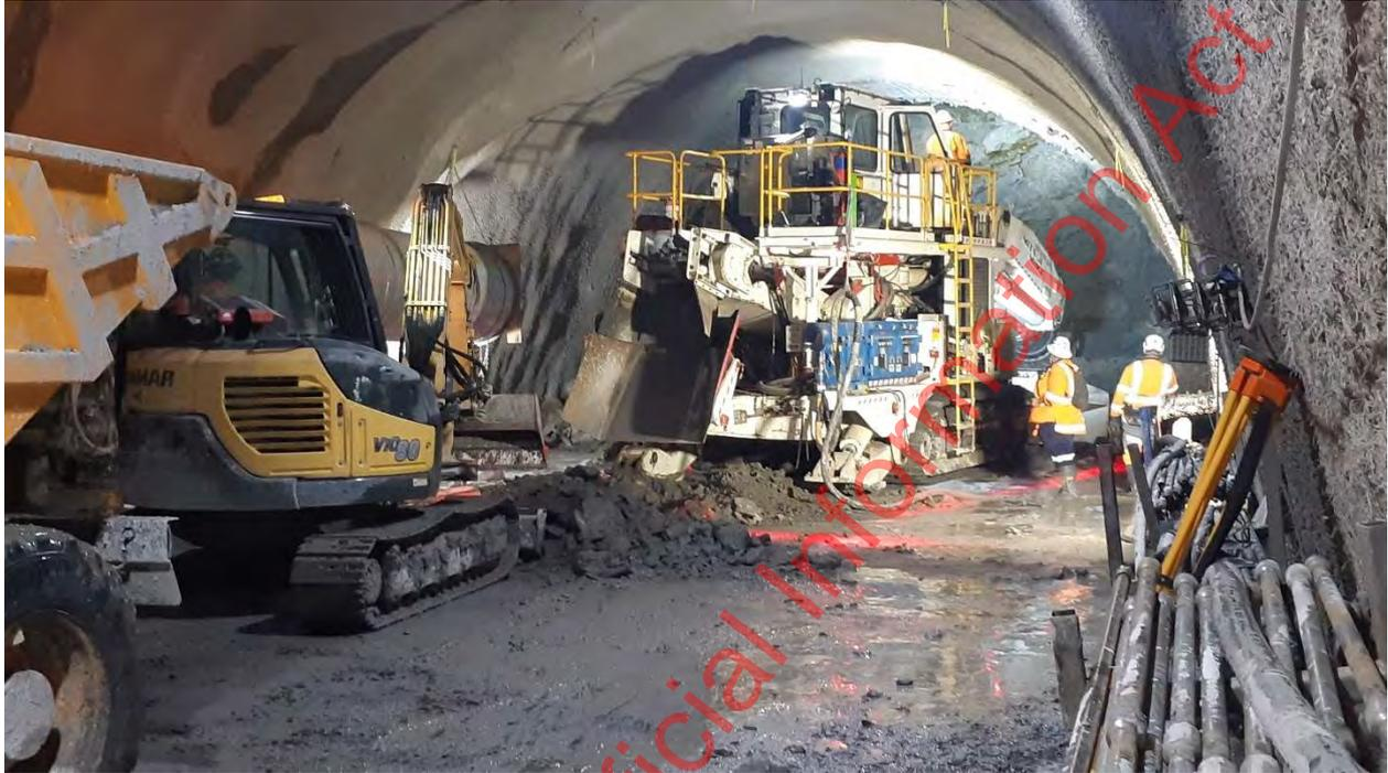
Figure 4 Mined Tunnel Construction, using a roadheader
