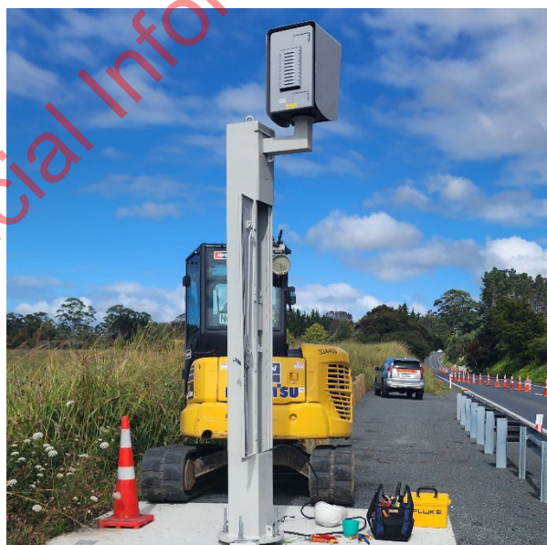
Figure 1: New pole being installed on the Matakana Road average-speed camera corridor near Warkworth
