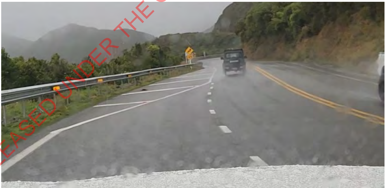
Figure 7: Continuity lines marked to end of Slow Vehicle Bay
