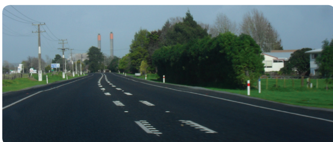
Wide centreline markings at SH1, Huntly, where passing is permitted
