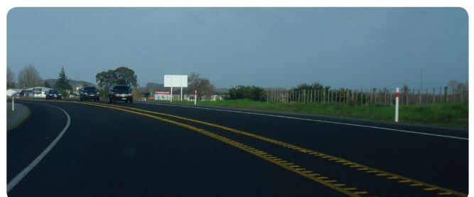
Wide centreline markings at SH1, Huntly, where passing is not permitted
