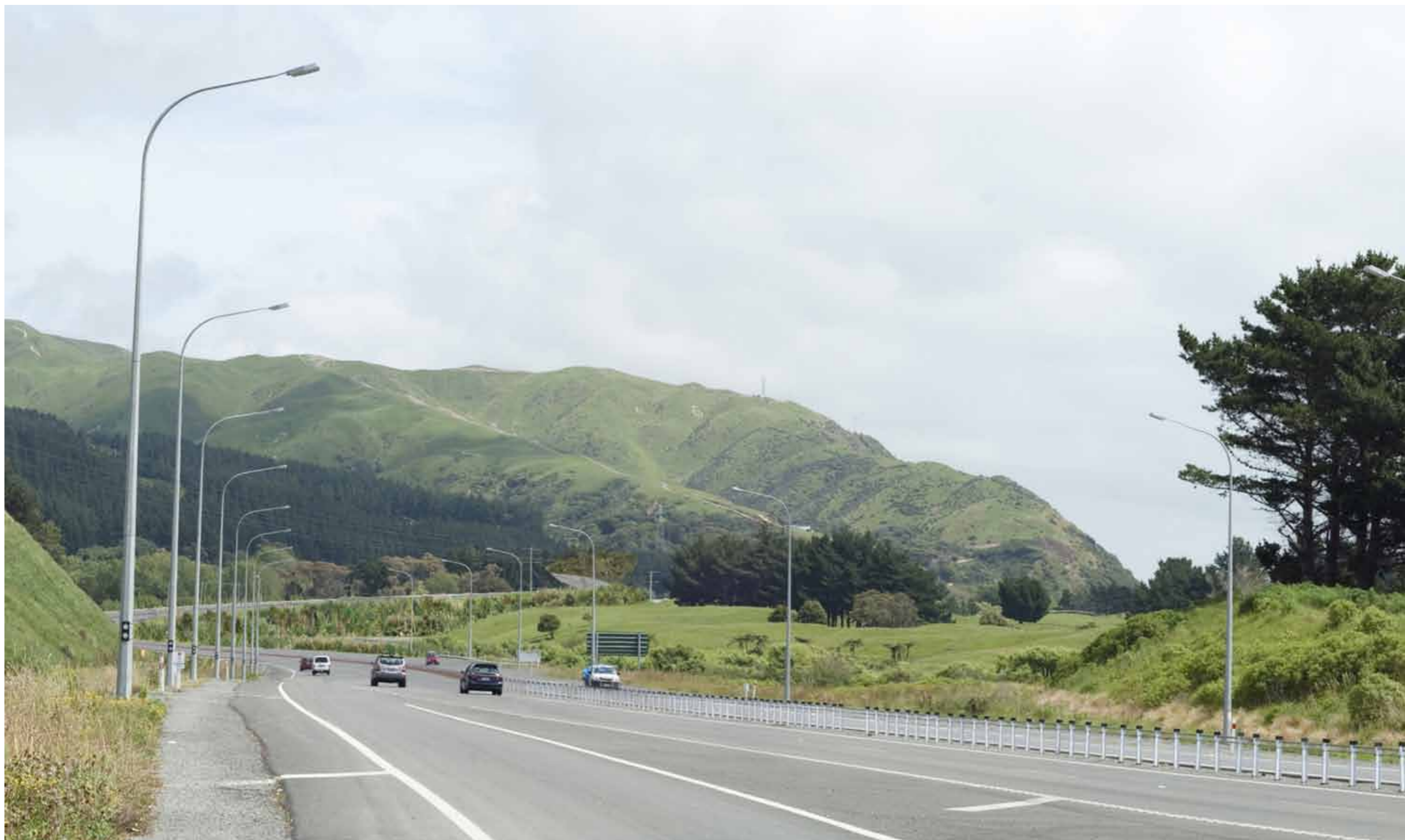
Figure 5.8: Looking south from southbound on-ramp at MacKays Crossing
