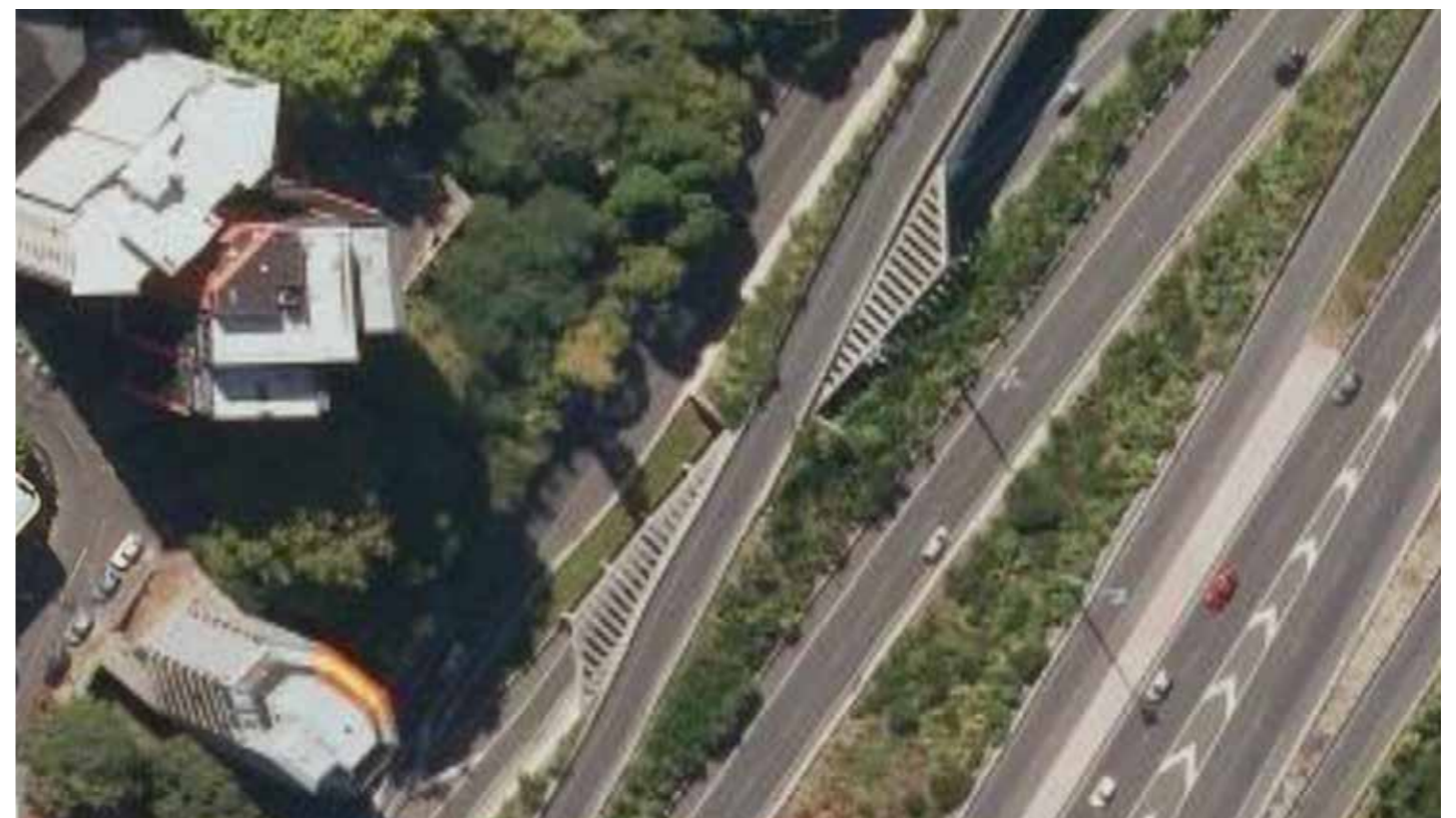
Figure 5.79: Grafton Gully structure similar to Bridge 27
